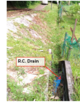
View 7 - Existing R.C. Drainage from Lot 21951
