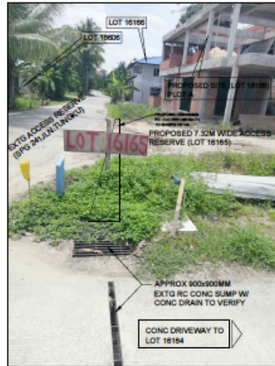
VIEW FROM LOT 18164 (EXTG CONC SUMP AND ROAD SIDE CONC DRAIN)
