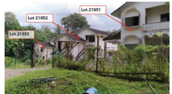
View 5 - Current Site Condition of Lot 21951, 21952 and 21953 showing the existing abandoned house to be demolished.
